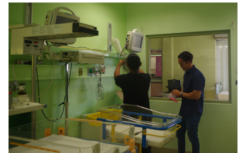
Biomedical technician and Andar technician during installation
